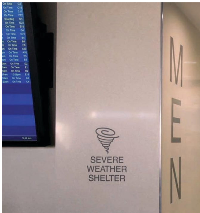
Figure 3-2. Sign for severe weather shelter integrated into finishes.
